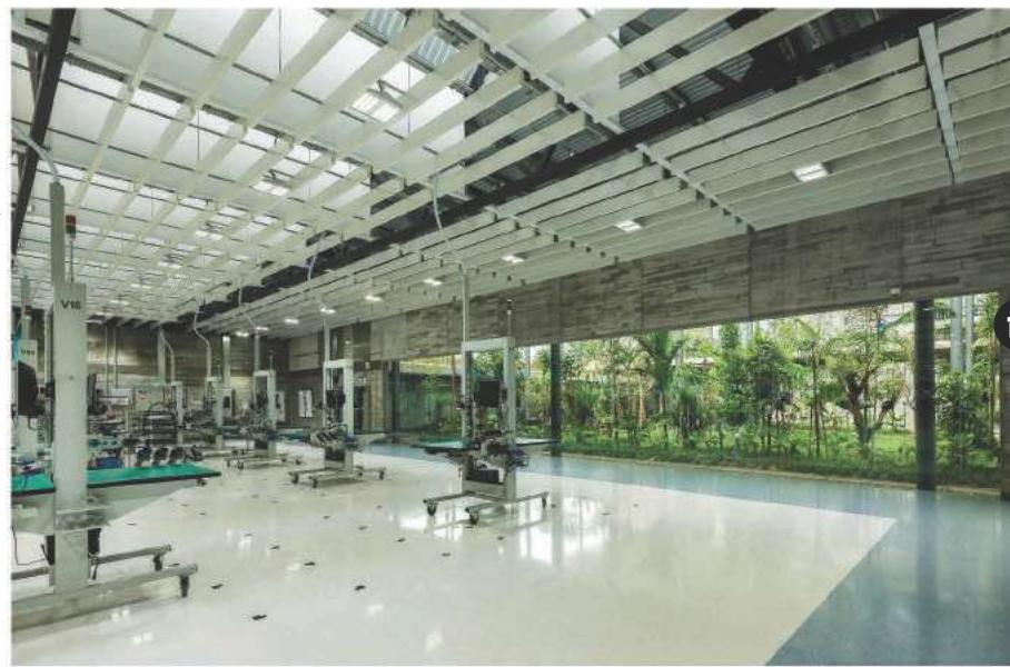
For the office block, the canopy louver roof was designed to provide effective solar protection from 2 pm onwards, i.e. during the hottest part of the day, while allowing streaks of sunlight through during the cooler morning hours. Pleasant diffuse evenly distributed daylighting for the entire factory production hall was ensured by North facing saw-tooth skylights.
